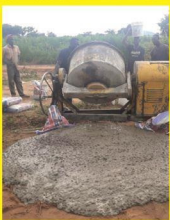
Casting of foundation for the ongoing fencing of ESN plot for National Secretariat at the University of Abuja
